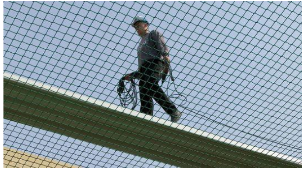
Figure 4: Typical safety net
