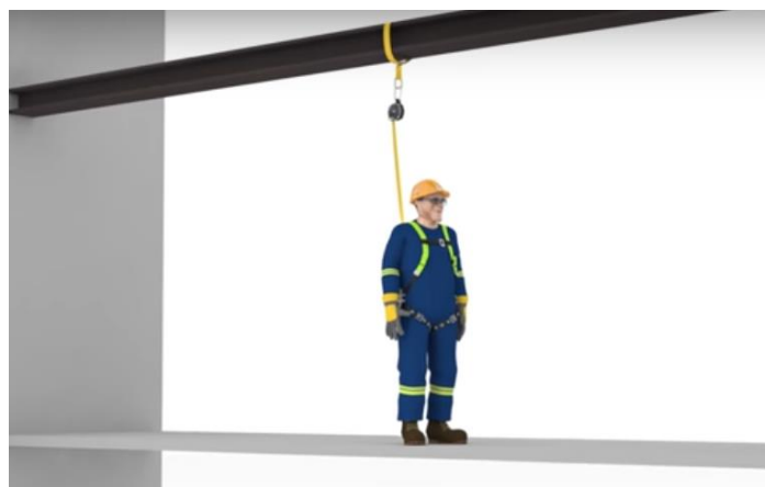
Figure 3: Safety harness connected to a self-retracting lifeline (SRL) with shock absorber
